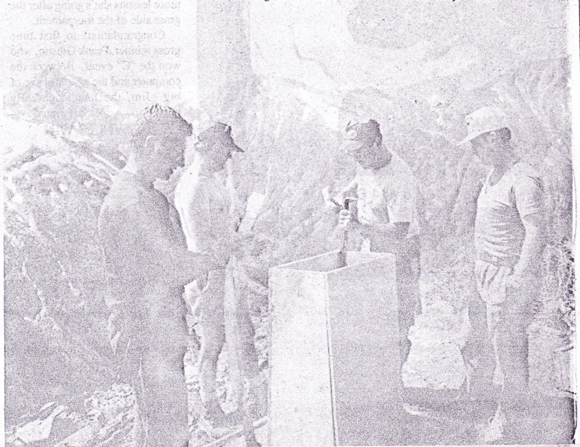
Cairn forms were prefabricated at Comox
