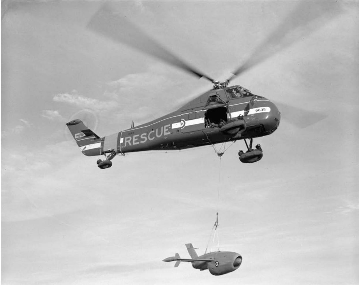
*Safely recovered from the lake, the KDA-4 Firebee is flown back to base slung underneath the helicopter - (RCAF Photo - PL-120088)*
