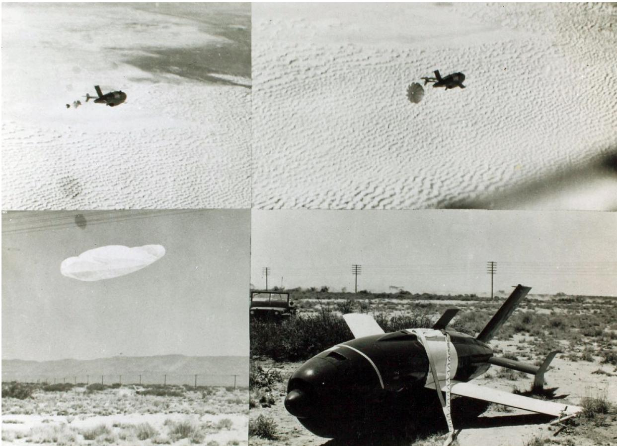
*The recovery sequence for the Firebee is shown in this series of photographs and the next. The recovery system was a two-stage parachute system; a drogue chute first slowed down the drone and then a much larger parachute deployed to lower the drone to the ground. - (Photo courtesy of the San Diego Air and Space Museum Archives)*
