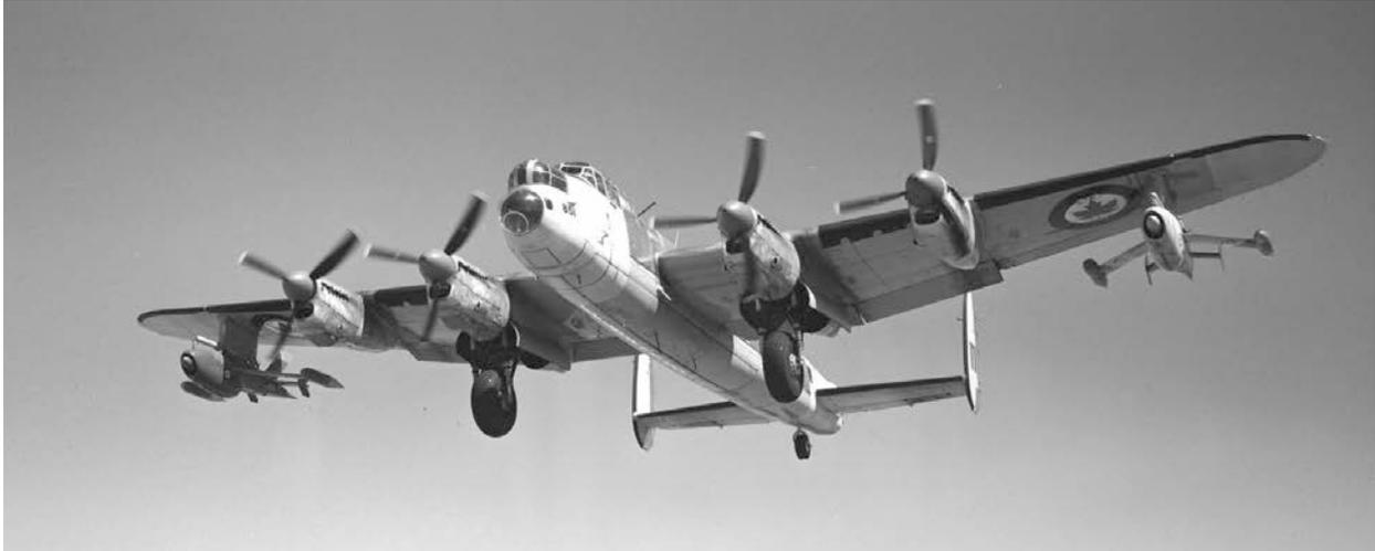
*Getting airborne for the mission, the drone controller Lancaster lifts off the runway carrying a Firebee under each wing tip - (RCAF Photo - PL-120072)*
