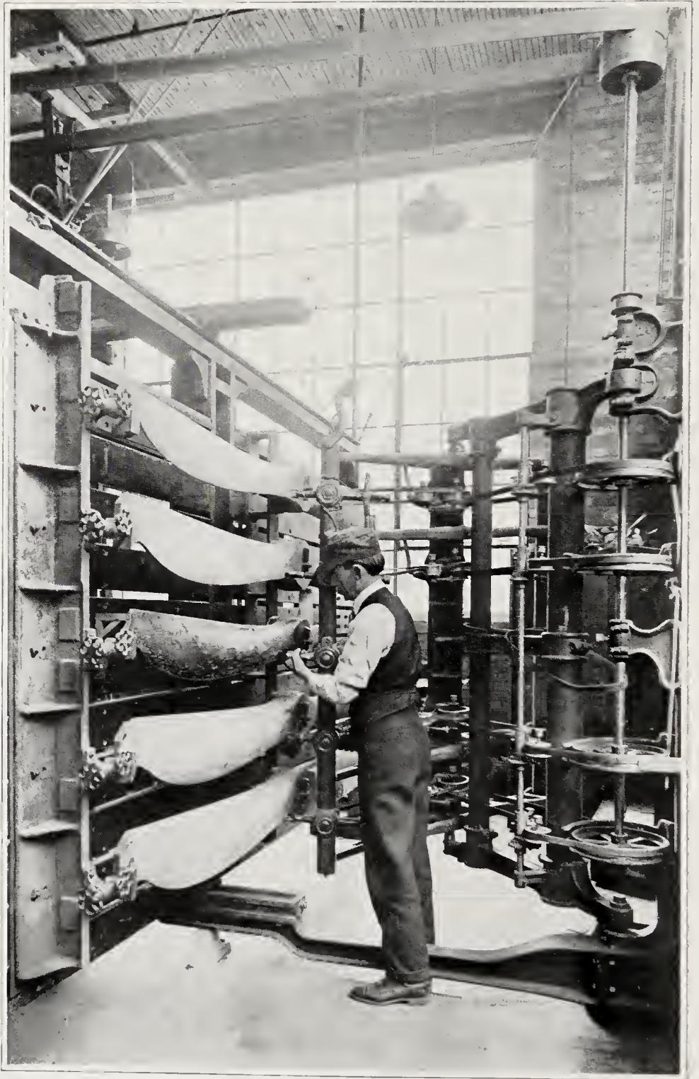
FINISHING PROPELLERS.
